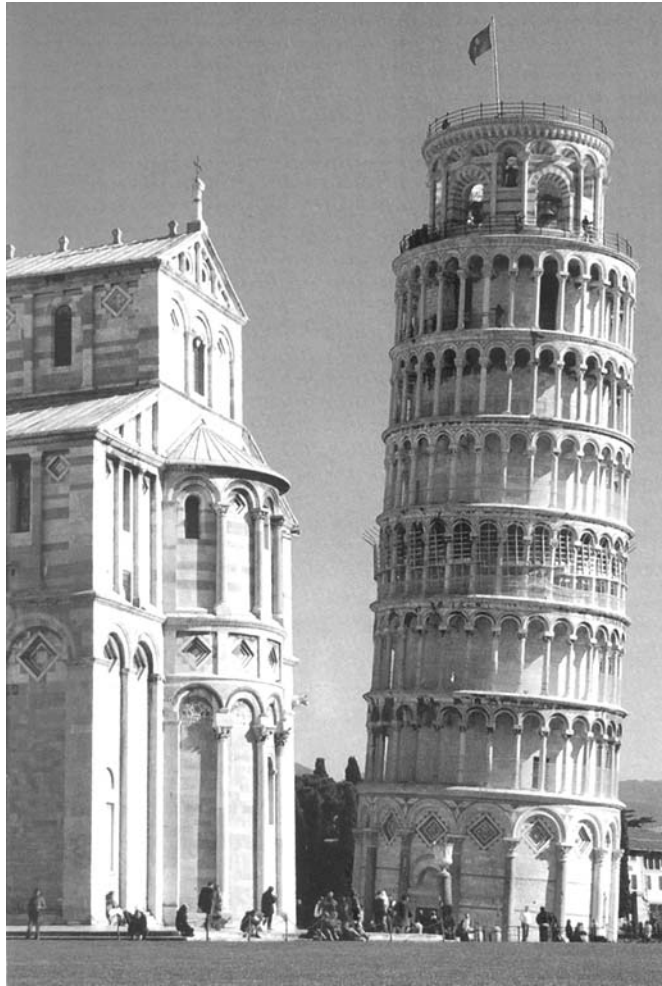
Fig. 1.1. The Leaning Tower of Pisa, Italy.
